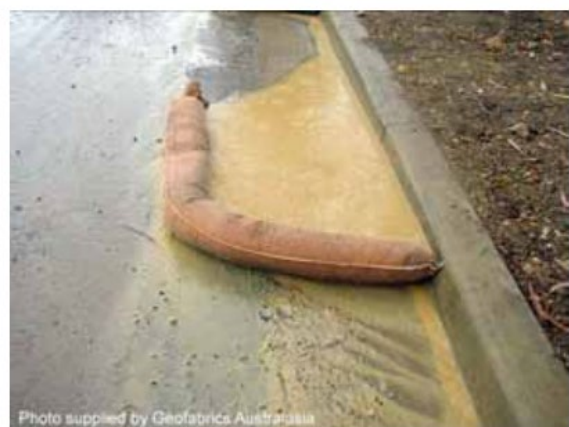
Filter sock sediment trap
