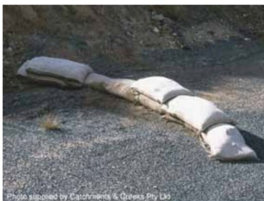
Sandbag sediment trap
