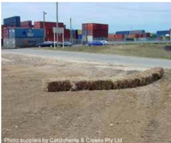
Straw bale flow diversion bank under construction (yet to be staked)
