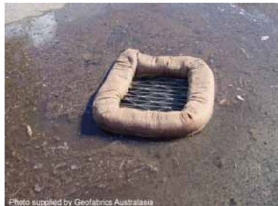
Filter sock drop inlet protection
