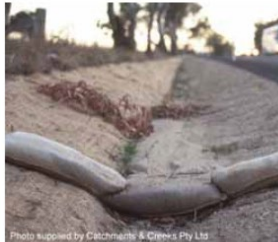
Sandbag check dam
